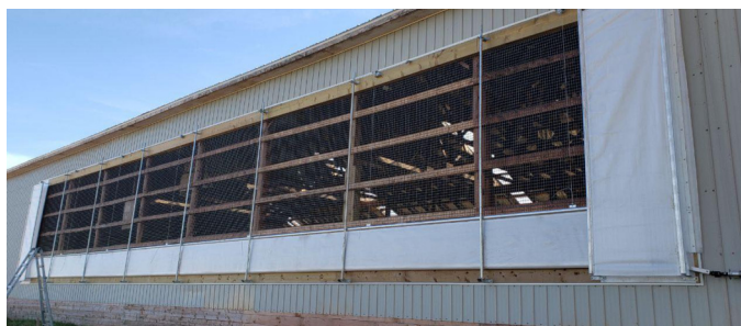
Faromor Roll-A-Way curtain system recently installed in western PEI.
