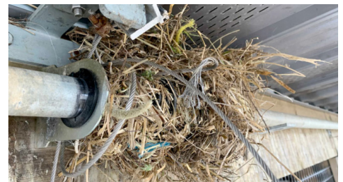
Bird nests can drip corrosive waste and get caught up in your cables, so be sure to remove them
