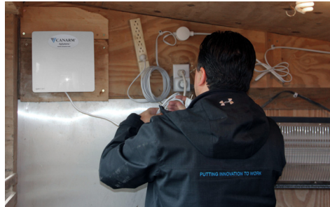
Poultry Products Manager, Nicholas Wilson installing a Breathe-Right HRV unit at a small flock Poultry barn
