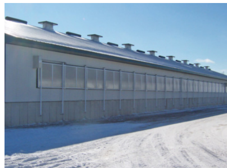
Natural ventilation system with clear panels on a barn are closed on a sunny winter day.
