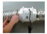
Attach the ducts with clamps.
