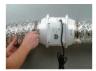
Attach the ducts with clamps.
