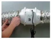
Attach the ducts with clamps.
