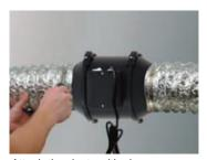
Attach the ducts with clamps.
