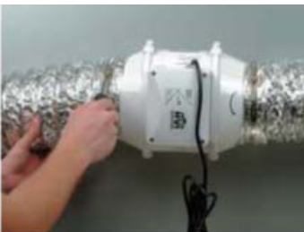
Attach the ducts with clamps.
