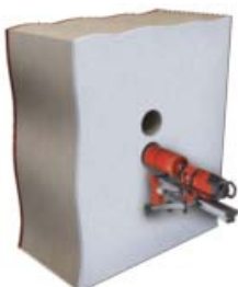
Drill the holes.
