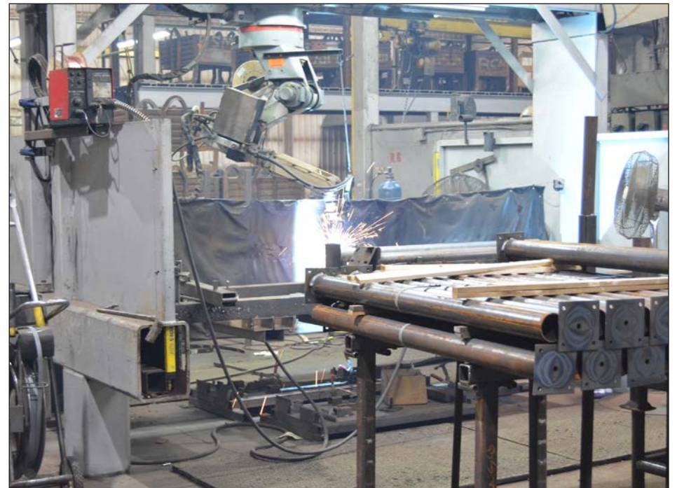
Motorman Robotic Welder. (2018)
